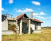
Manager's Office, Waipaoa Freezing Works, Outside Gisborne, 2016 Archival pigment print 715 x 875 mm framed Edition 1 of 7 $3,400 (framed, UV glass)
