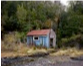
Winter, Powerhouse at the Old Escarpment Mine, Denniston Plateau, 2016 Archival pigment print 715 x 875 mm framed Edition 3 of 7 $3,500 (framed, non reflective UV glass)
