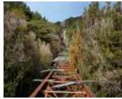
Bridge at Middle Break, Denniston Incline (After Lock), West Coast, 2016
