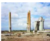
Kilns and Tanks, Demolition of the Cement Works, Cape Foulwind, West Coast, 2019 Archival pigment print, conservation framed with ash wood, museum glass 1100 x 1350 mm ed 1/7 $8,200
