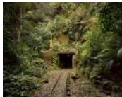
George's Tunnel, Waitākere Dam Tramline, 2015 Archival pigment print, conservation framed with ash wood, museum glass 920 x 1135 mm ed 1/7 $6,000 (framed)
